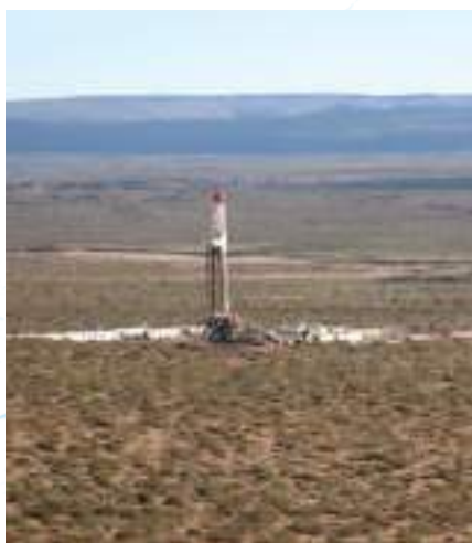
Drilling tower in Rincón la Ceniza. © Ike Teuling
